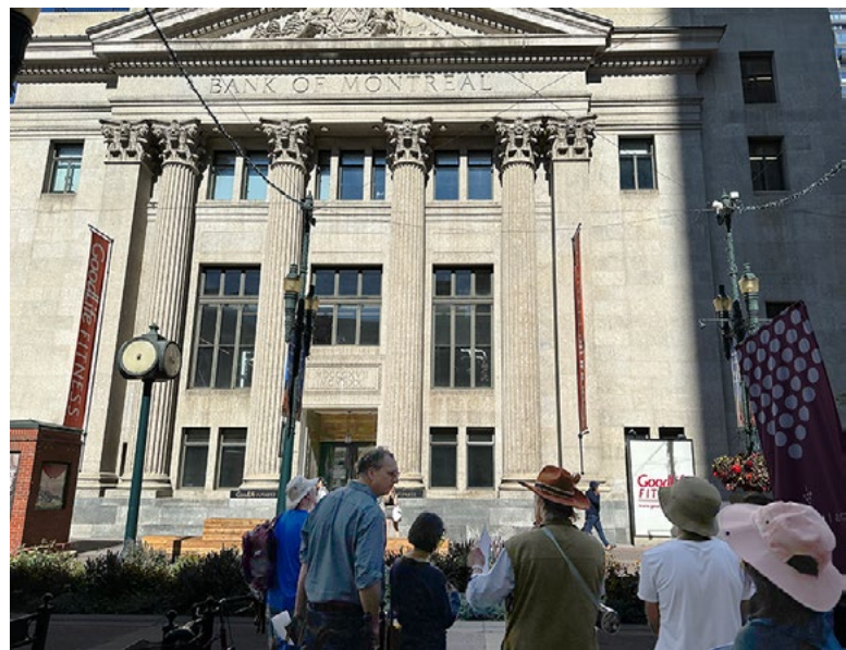
Figure 5. The Bank of Montreal building, showcasing the beauty of Tyndall stone. Despite decades of weathering, the carvings are still extremely detailed. Photo: Eric Campbell.
